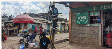
FIBRE BUILD, KENYA
